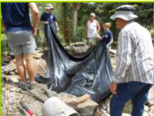
Master Gardener Tony Donzello (photo center) with Rotaract volunteers relining the Extension Horticultural Learning Center Gardens water feature.
