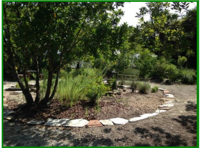
New planting bed under construction
