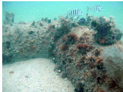
Culverts such as these are often deployed in small piles to allow adequate spacing between the structures; such layouts help increase the overall production of the reef site.
